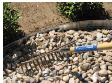
5. Backfill 1/2' below edging
